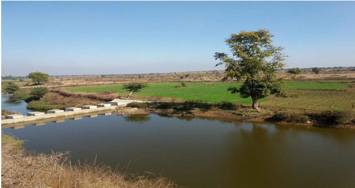
Stop Dam Constructed Under BRLF EU program at Kalothara village
